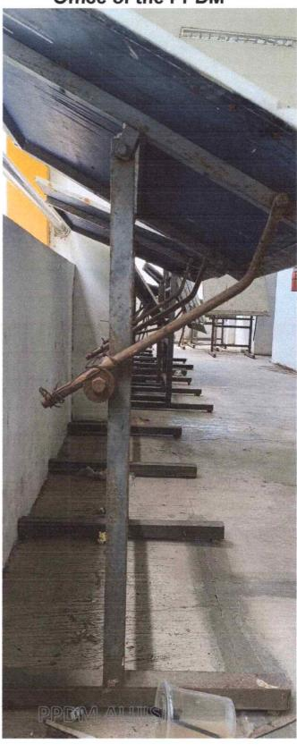
FINDINGS: -Defective Board -Rusted Board Lifter -Loose and Tight Screws
